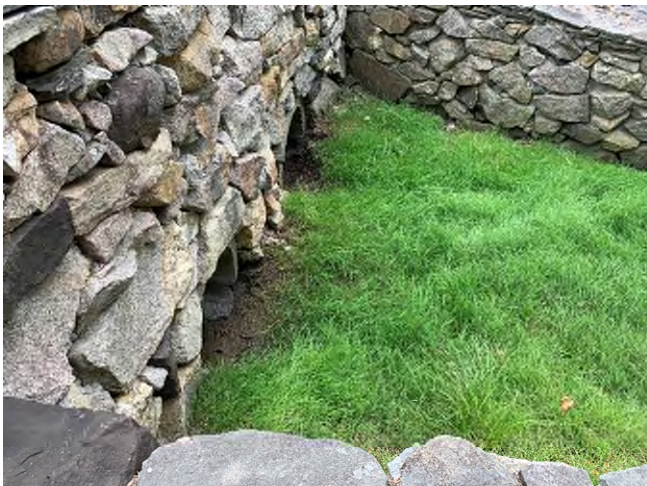
4 Brickyard Circle - 1 (Drainage Course)
