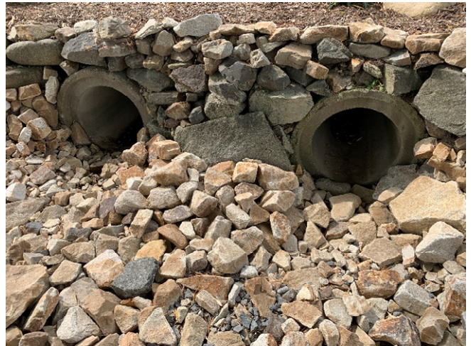
64 Gundalow - 2 (Drainage Course)
