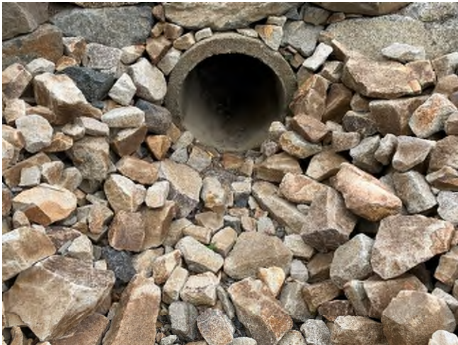
64 Gundalow - 1 (Drainage Course)
