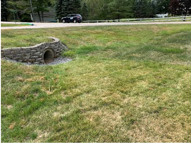
29 Gundalow -1 (Drainage Area)
